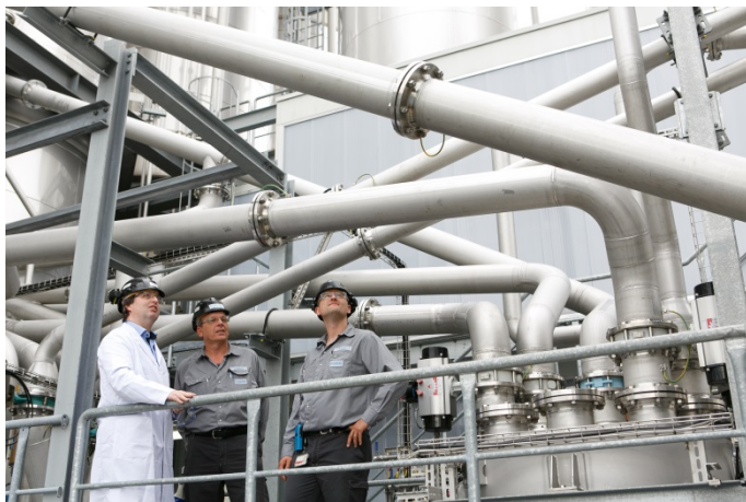
[Photo 3] Energy-saving transport to the silo: An interdisciplinary team at Kuraray is committed to making facilities and processes at the company's production sites more efficient. One example is improved networking of the high-pressure conveyor system at Höchst Industrial Park that transports powders and granulates from the Mowital® and KURARAY POVAL™ production facilities via pipes between process steps and to the silos used for interim storage. The energy required for this has been reduced significantly by improved networking of the compressors.
